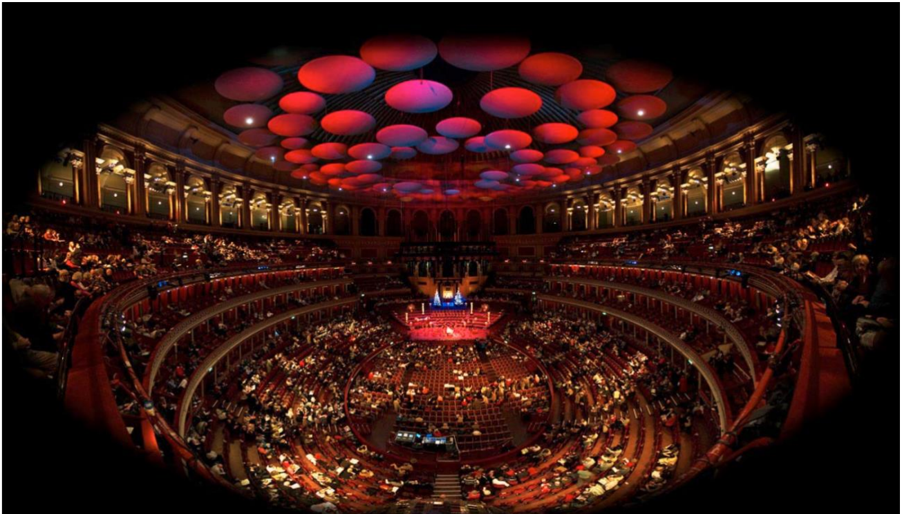
Figure 15: The Royal Albert Hall, London: Large fibreglass acoustic diffusing discs in the roof remove the echo from the Albert Hall. Prior to their installation in 1969, it was said that the hall was the only place where a British composer could be heard twice.
